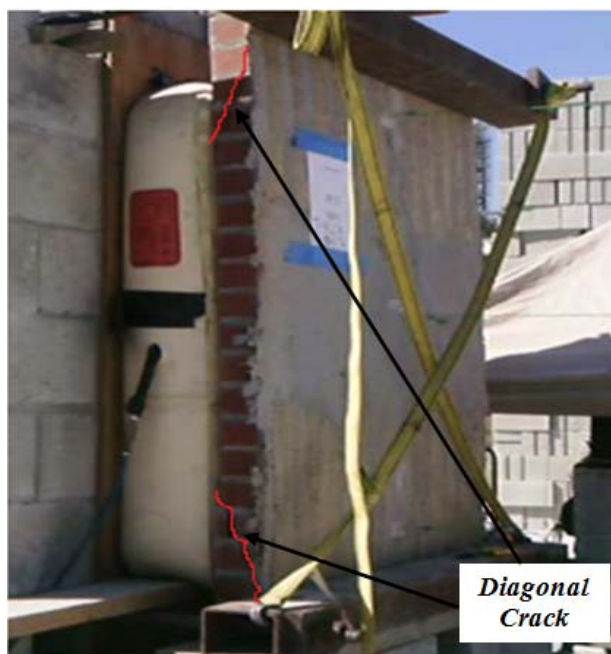
(f) (Enhanced crack lines)
